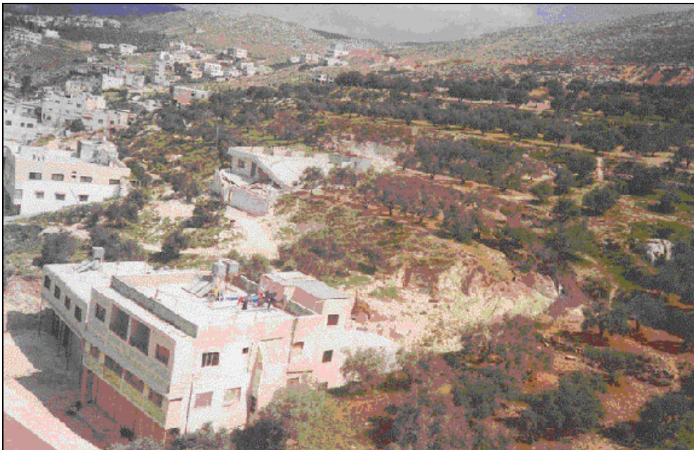
Figure (3): A Photograph shows the Landslides and the damaged house in
